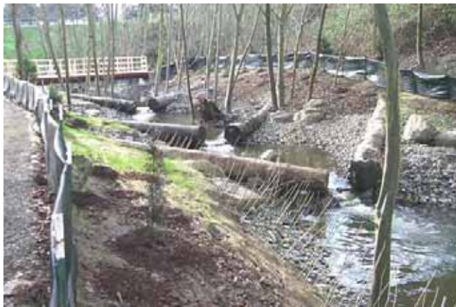
Completed Longfellow Creek, a project of Seattle Public Utilities.
