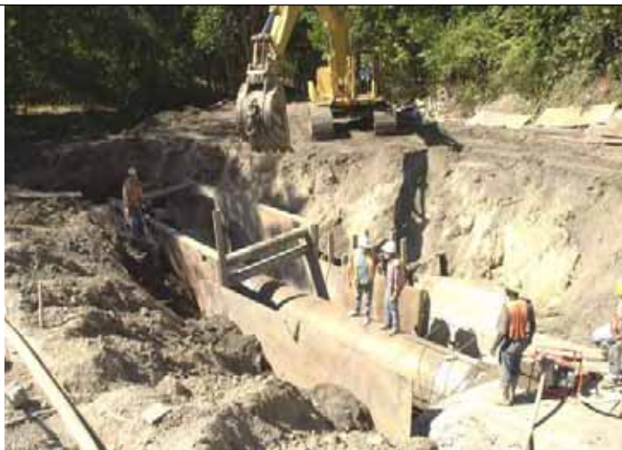
Long Fellow Creek Construction
