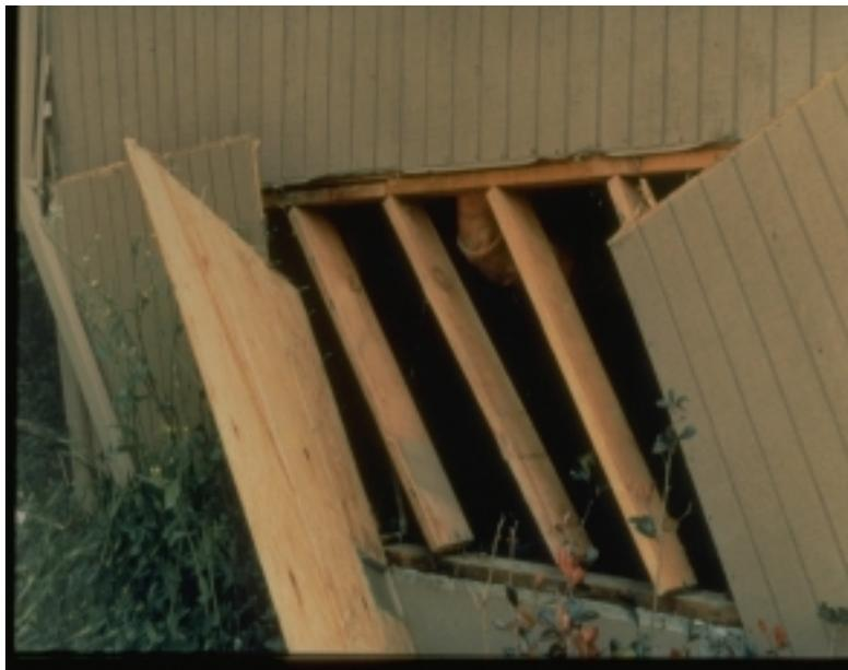
**Figure 4. Collapse of the short wall between the first floor and the foundation (photo from Applied Technology Council)**
