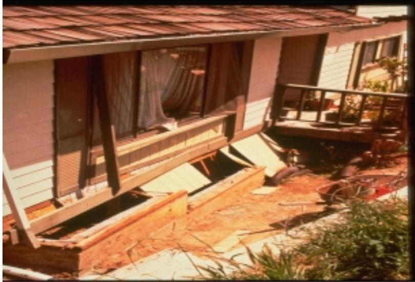
**Figure 3. Home moved off the foundation wall (photo from Applied Technology Council)**
