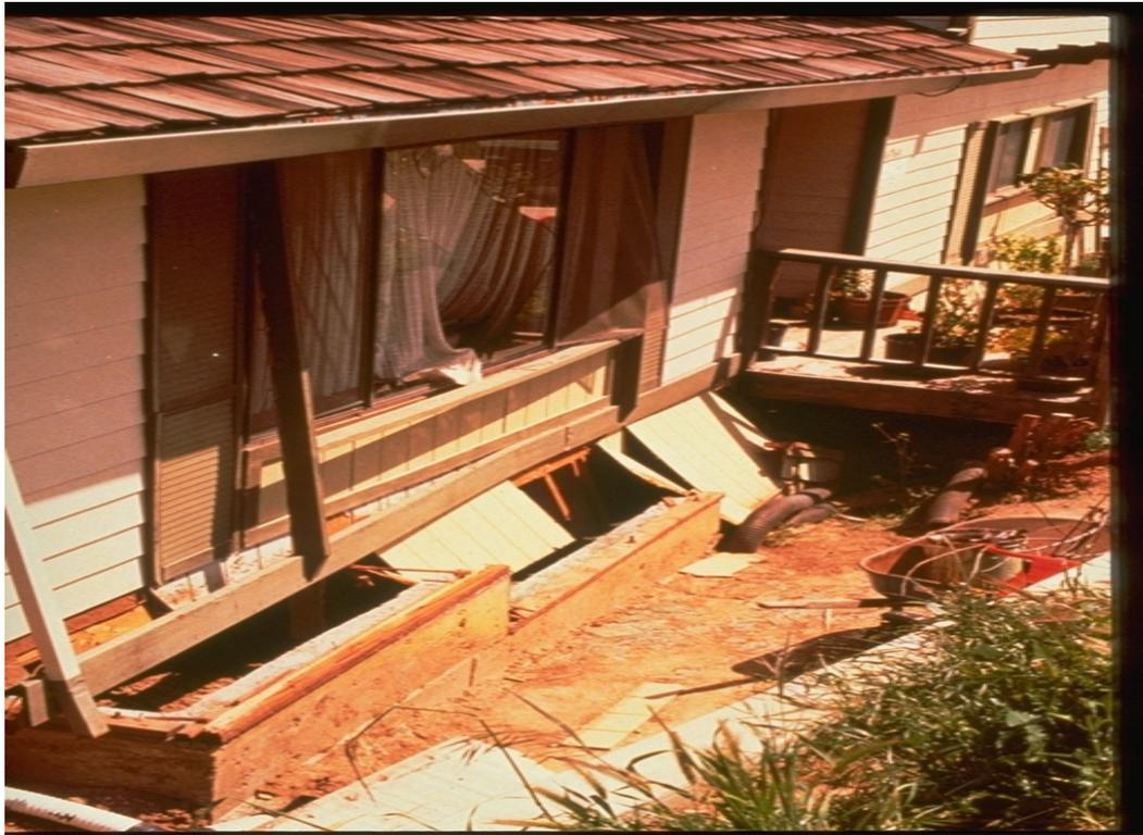
**The Standard Home Earthquake Retrofit Plan is limited to wood-framed single-family homes and multiple-family buildings with fewer than four dwelling units. The standard plan is not a suitable strengthening method for all homes. Review plan qualification criteria to determine if you may use this plan.**
