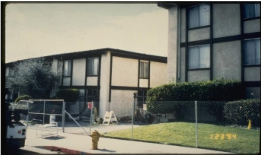
**Figure 6. Collapse of apartment building with weakened first floor. The apartment on the left was a three-story building (Photo by Eugene Trahern, Coughlin Porteer Lundeen)**
