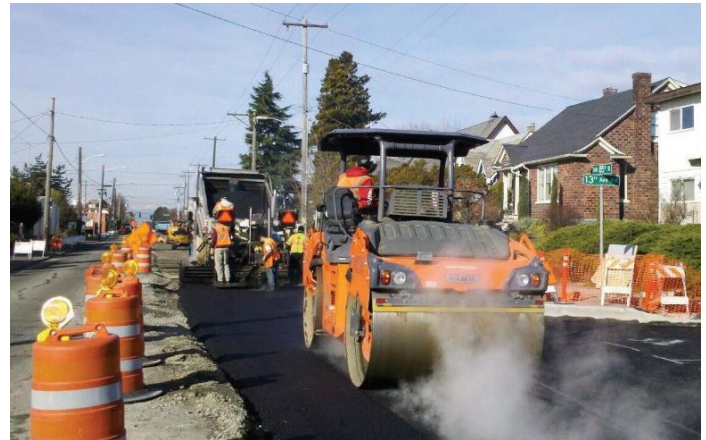
Example of crews paving the street
