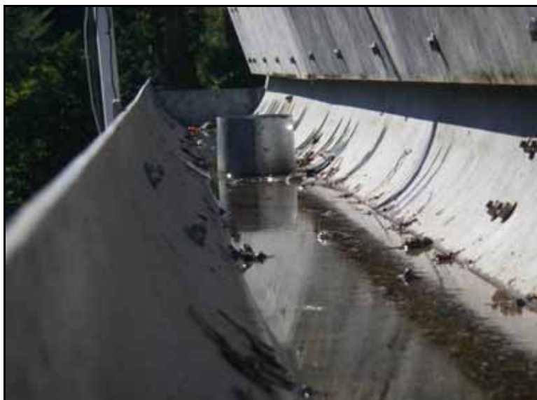
Figure 2-2 Downspout Risers Installed in the Roof Gutter
