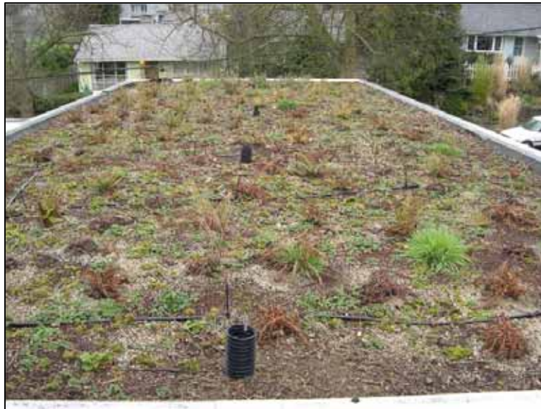
Figure 2-12 Green Roof located on the East Roof of the Shelterhouse
