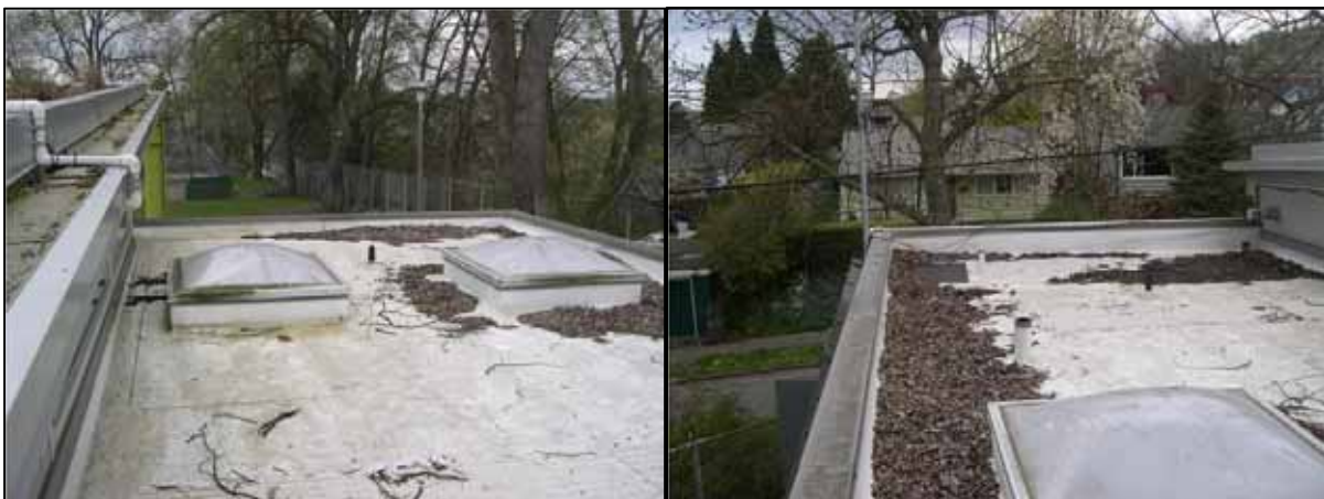
Figure 2-11 Conventional Roof Located on the West Roof of the Shelterhouse
