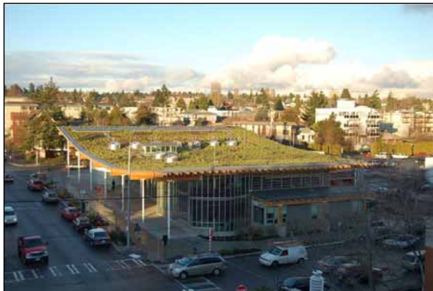
Figure 2-6 Green Roof on the Seattle Public Library Ballard Branch
