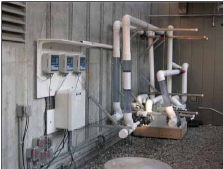
Figure 2-17 FS10 / EOC Flow Monitoring Station Located on the West Side of the EOC Building
