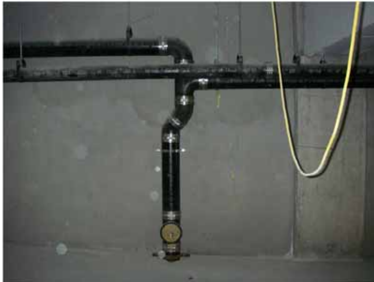
Figure 2-20 Location of the SCPG Main Flow Monitoring Station on Level P2
