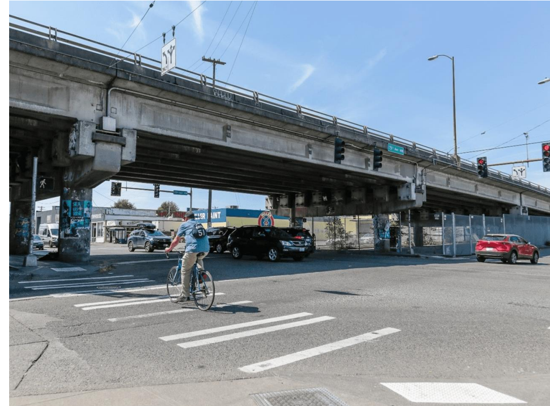
15 th Ave NW/Leary Way Bridge
