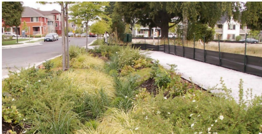
A completed natural drainage system.
